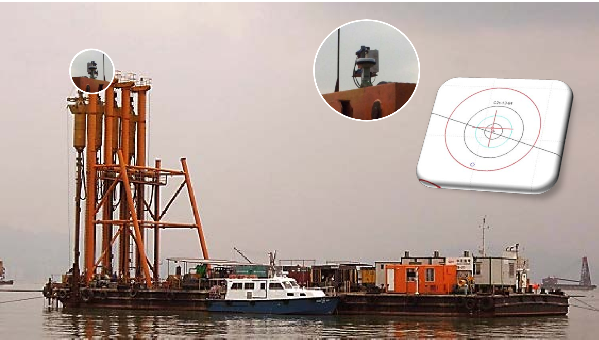
Barge for the installation of stone columns
